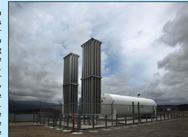
Casitas Municipal Water District installed a new hypolimnetic oxygenation system during September of 2015 to help minimize water quality problems in Lake Casitas.
